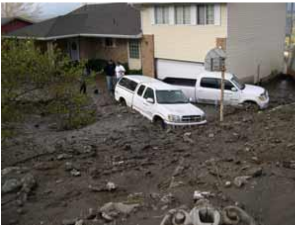
House damaged by the April 6, 2004 debris flow in Farmington, Utah.
